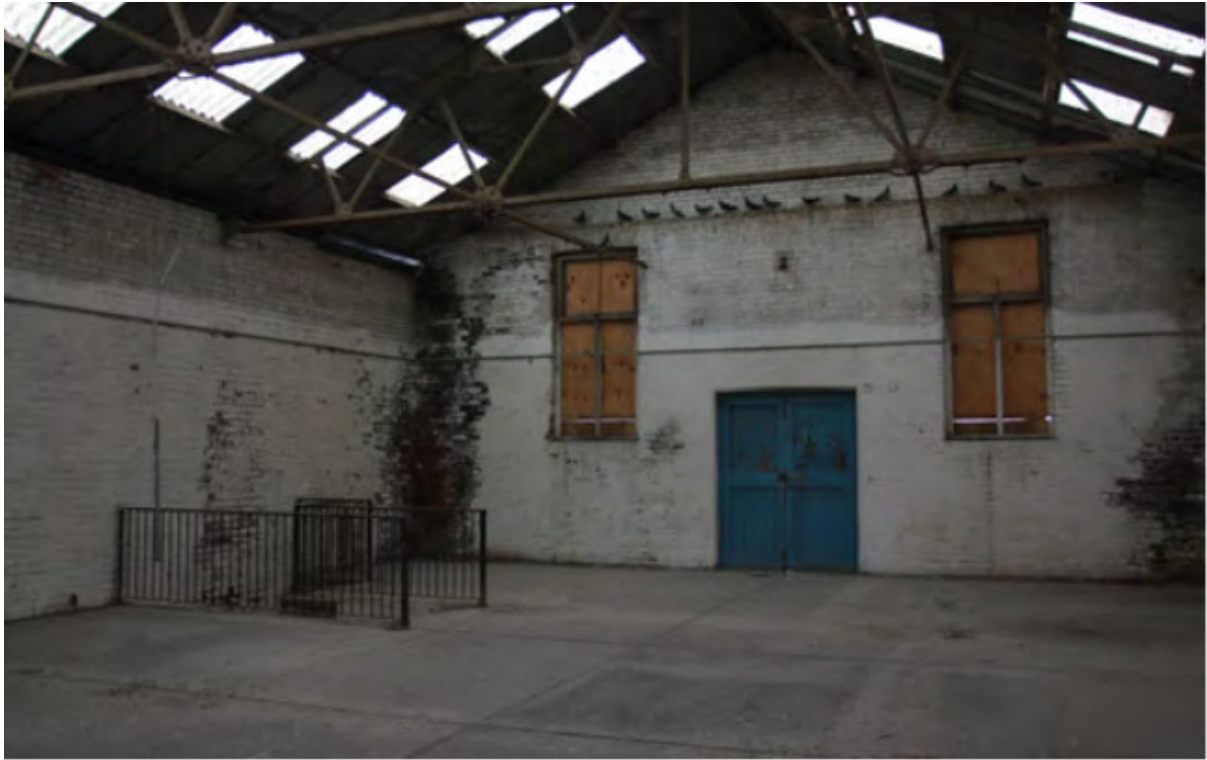
Boiler House Upper Level interior 2016
