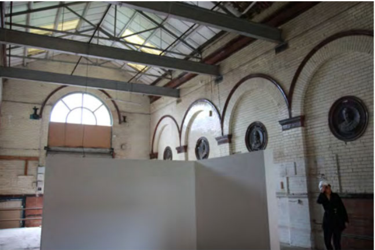
Engine House interior 2016
