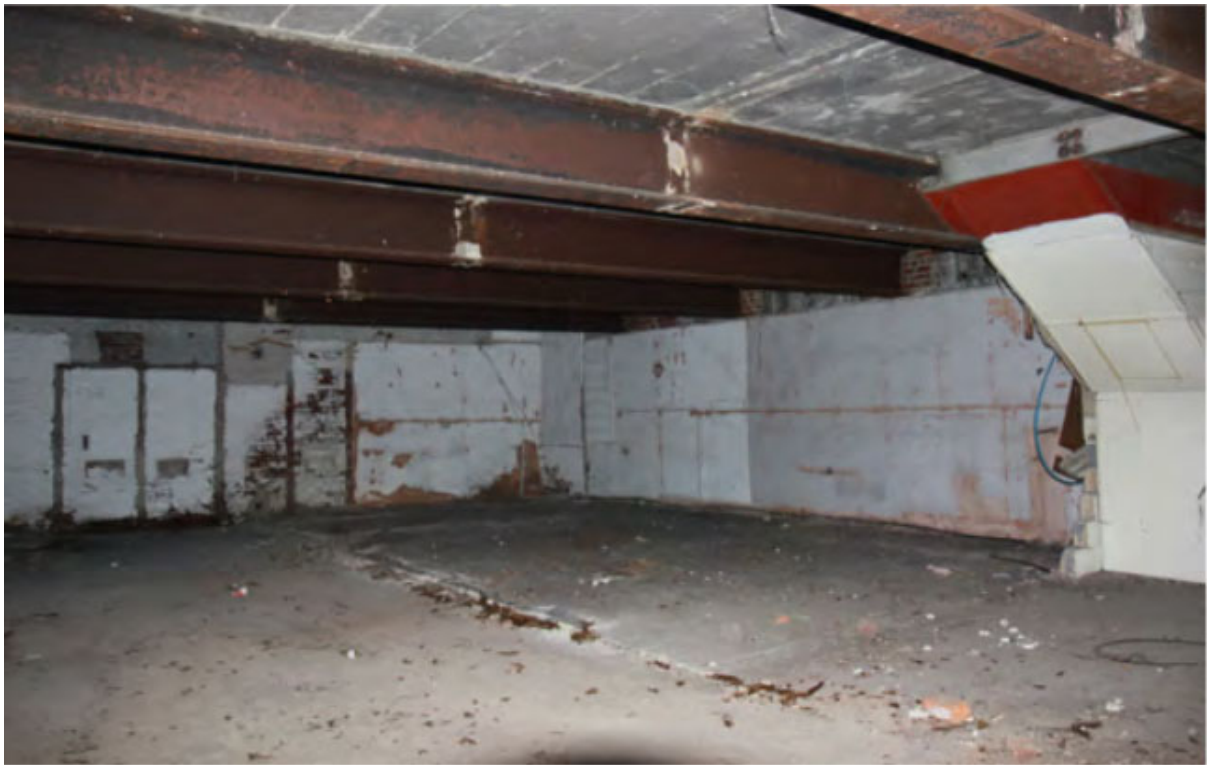
Boiler House Ground Floor interior 2016
